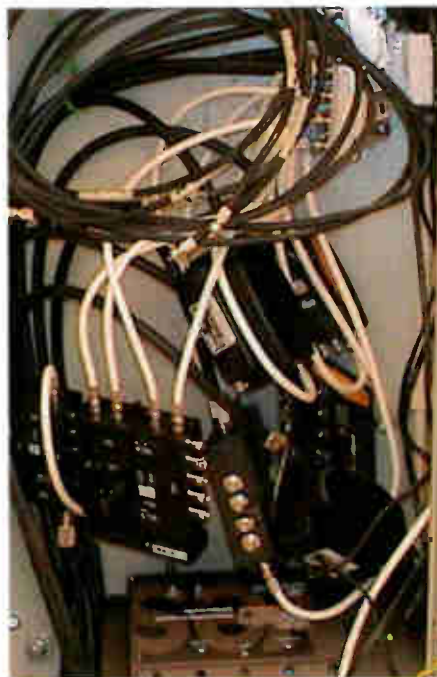
Photo 1: Part of a poor satellite distribution system that had to be rebuilt.
